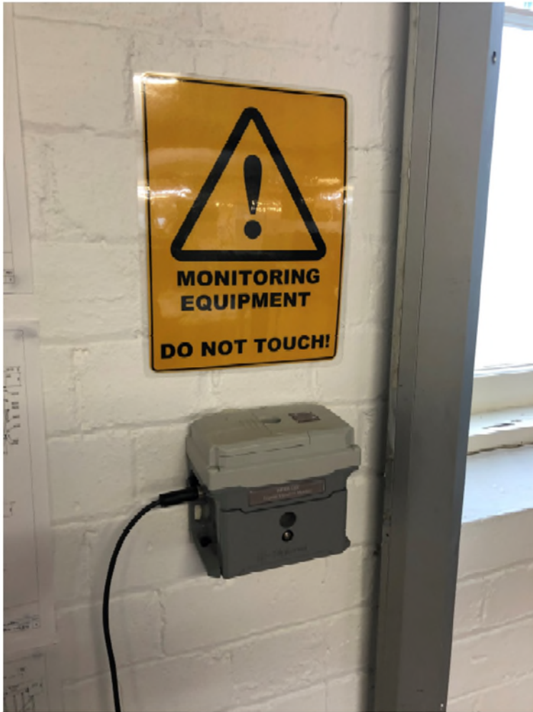
Figure 5-2 - On site real-time vibration monitor at 25 Hickson Road
