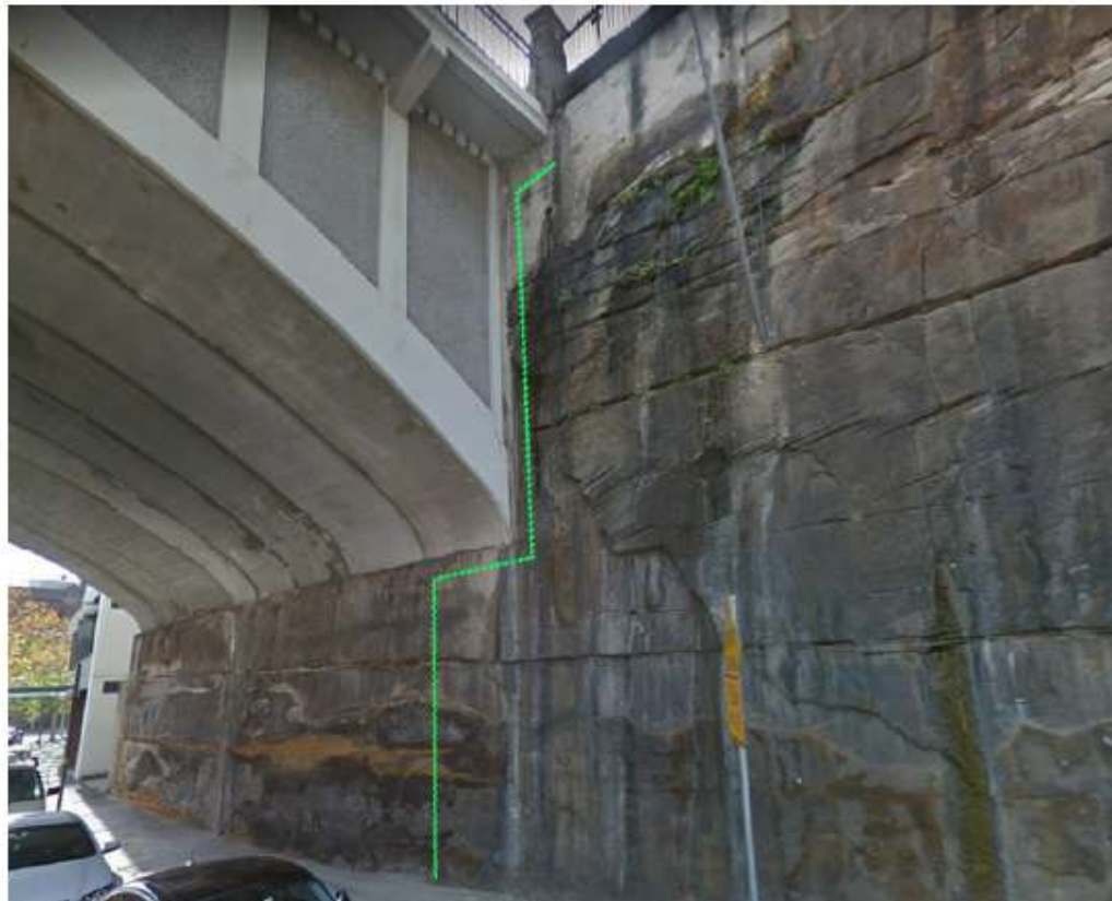
Figure 5 Proposed location of the gas diversion shown on a Google Street View capture taken in October 2014, before the acoustic shed was constructed. The Windmill Street bridge is at the left.
