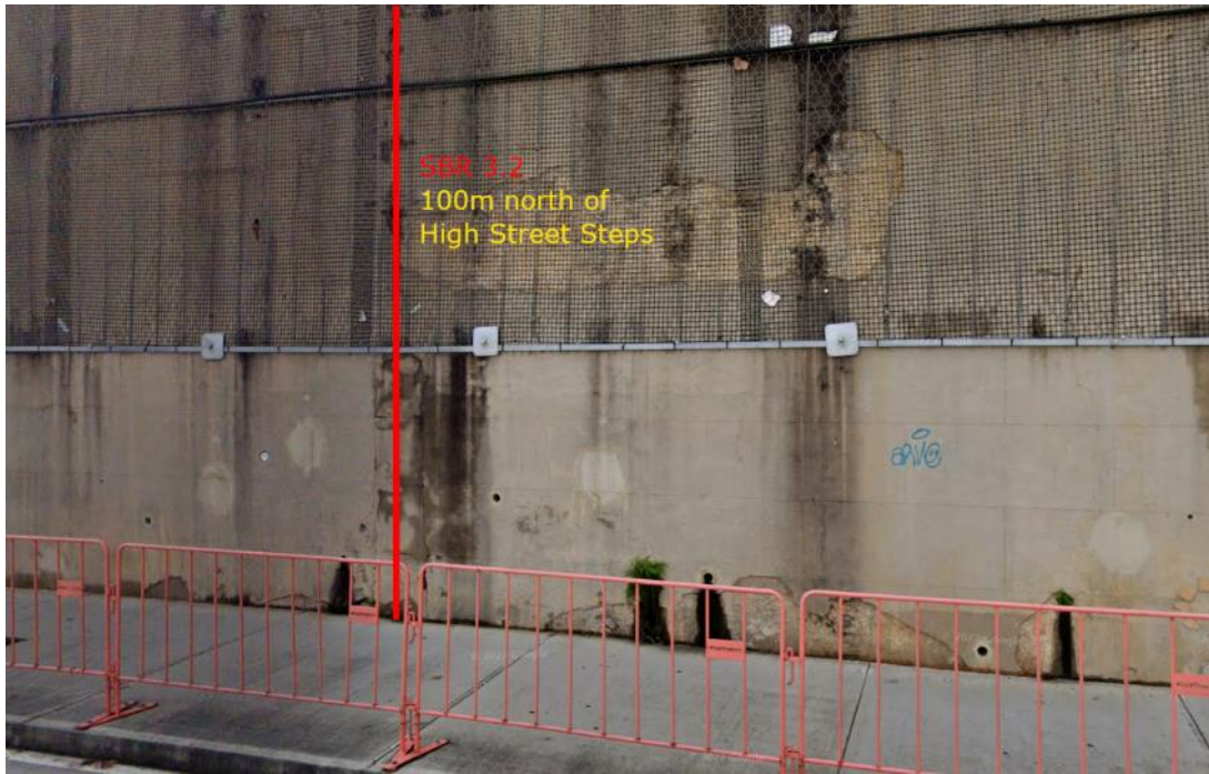
Figure 3: Location of downpipe SBR 3.2.
