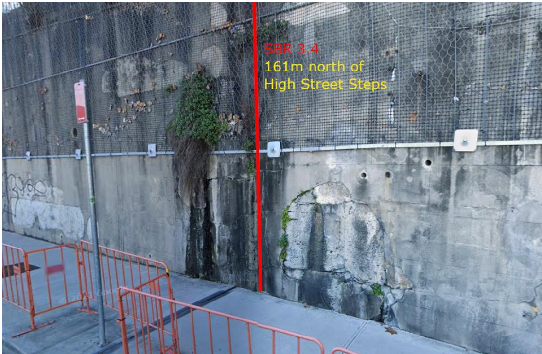
Figure 5: location of downpipe SBR 3.4.
