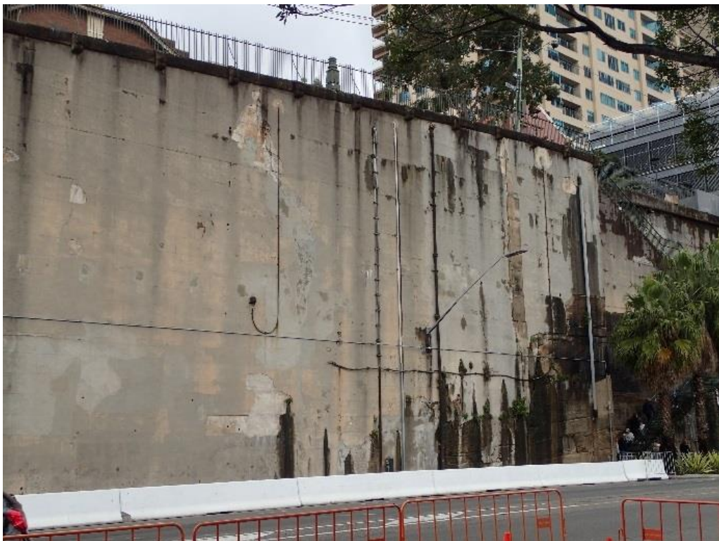
Figure 14: A collection of existing services attached to the wall.
