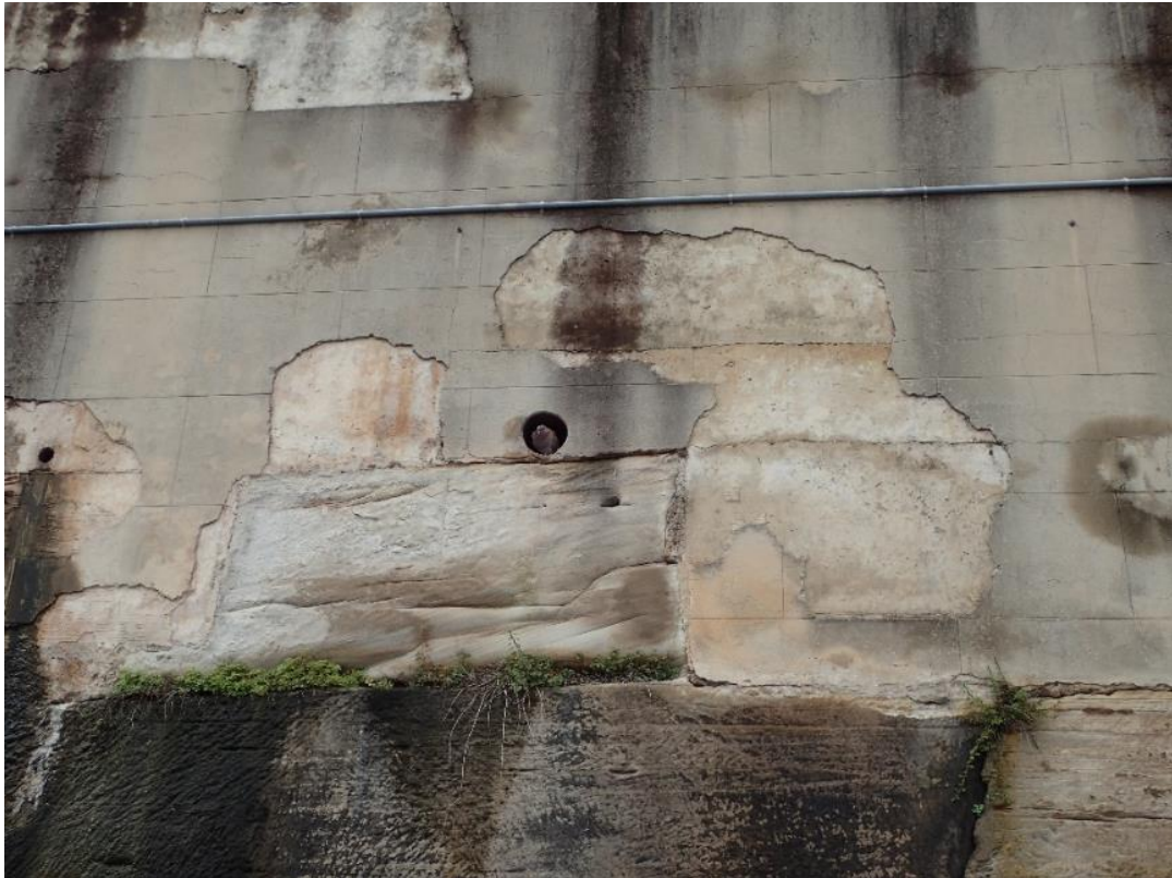
Figure 11: A section of the cutting and wall. The render is scored to replicate masonry blocks and is aligned along the line of the natural bedrock, above which the underlying sandstone blocks have been exposed.
