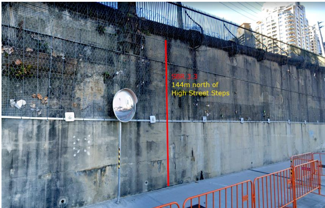
Figure 4: Location of downpipe SBR 3.3.
