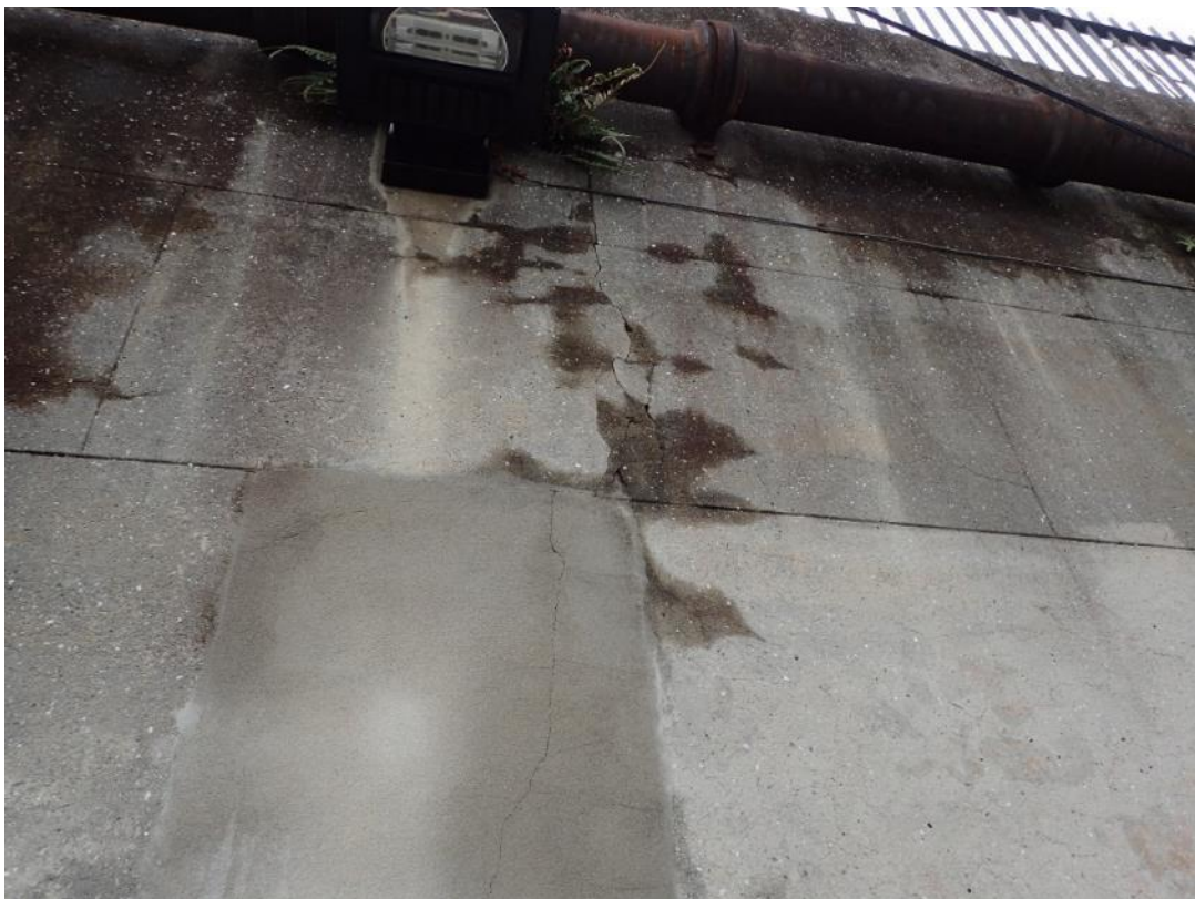
Figure 12: A patch of modern cement render surrounded by the original render. The white flecks are shell fragments.
