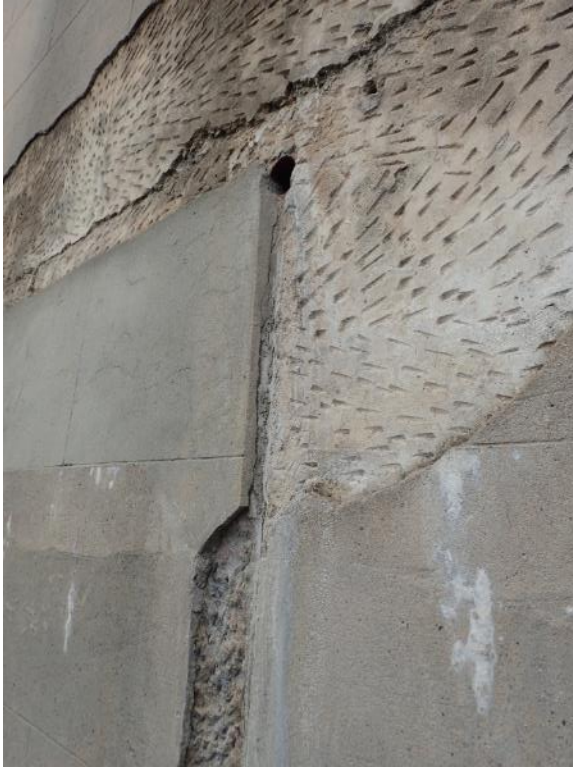
Figure 13: Exposed patches of render indicate that at least some sections have three layers of render and the lower layers are pecked to create a rough surface for the next layer.
