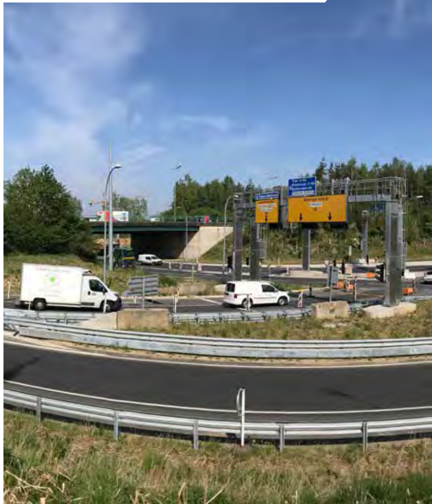
IRRGARTEN (SCHAFFNER) ROUNDABOUT - LUXEMBOURG
